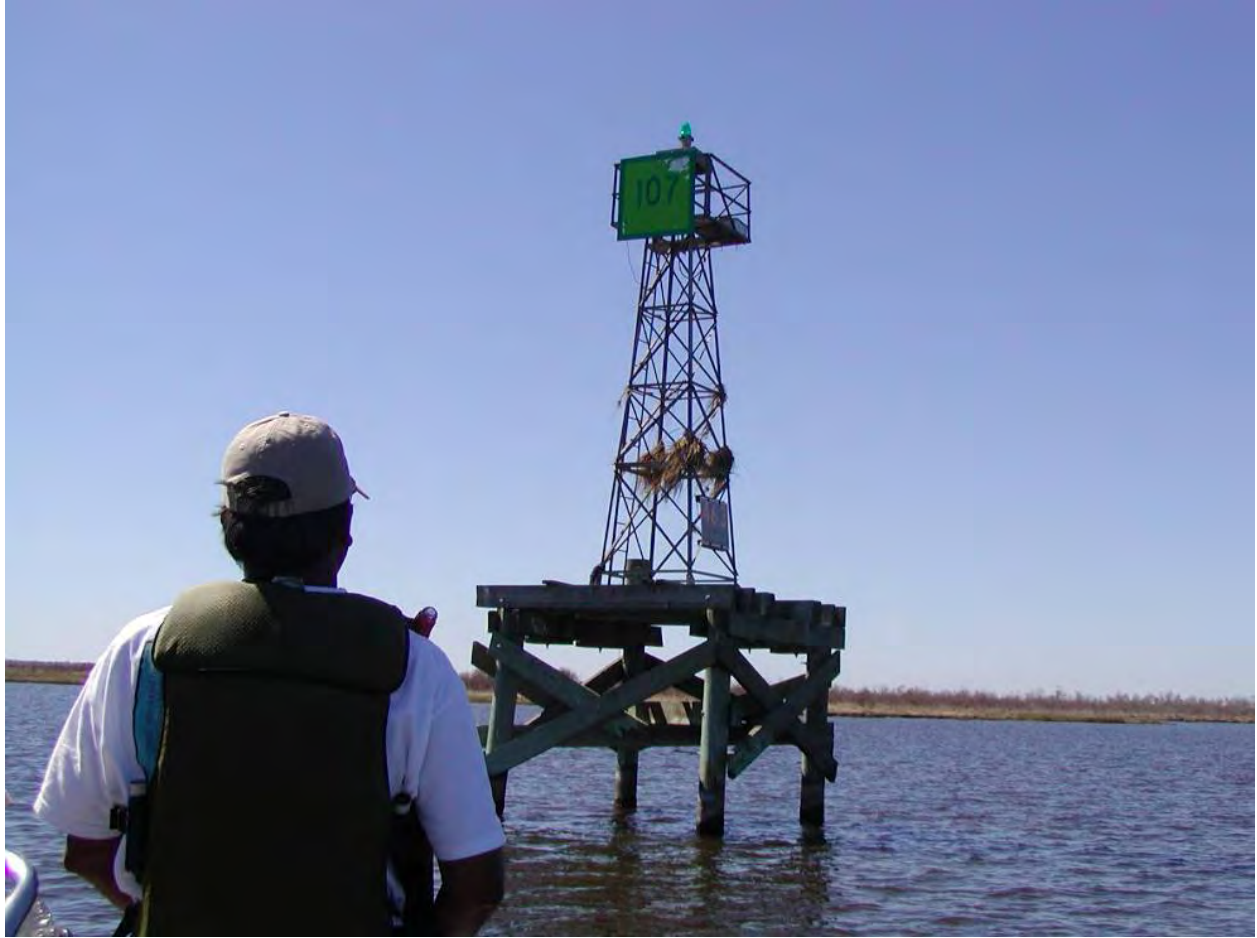
Figure 20. LA 1155 on MRGO. Debris on tower
