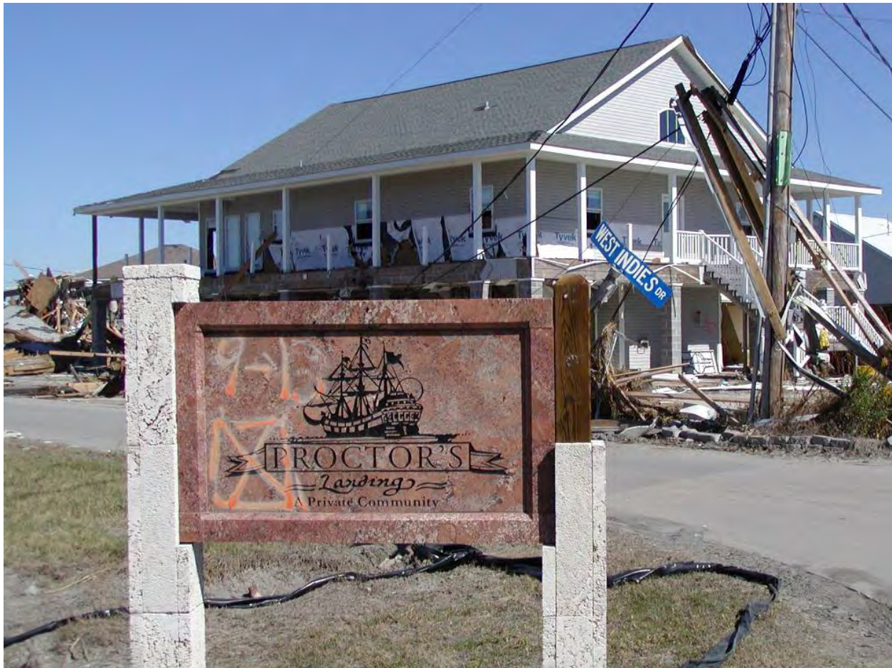
Figure 21. Home in Shell Beach containing high water mark LA 1087 at 31" above second level floor.
