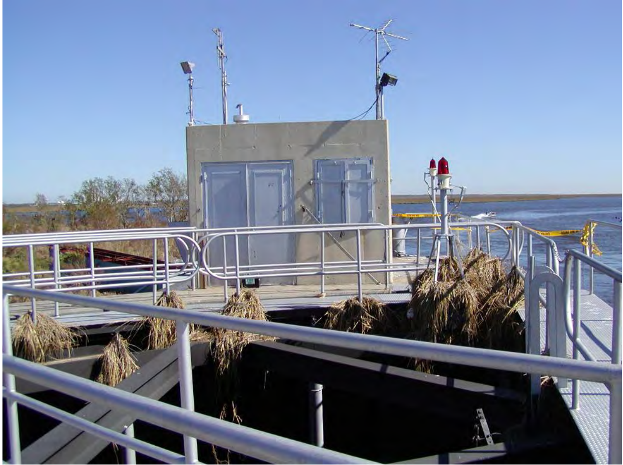
Figure 19. Bayou Bienvenue Gauge House
