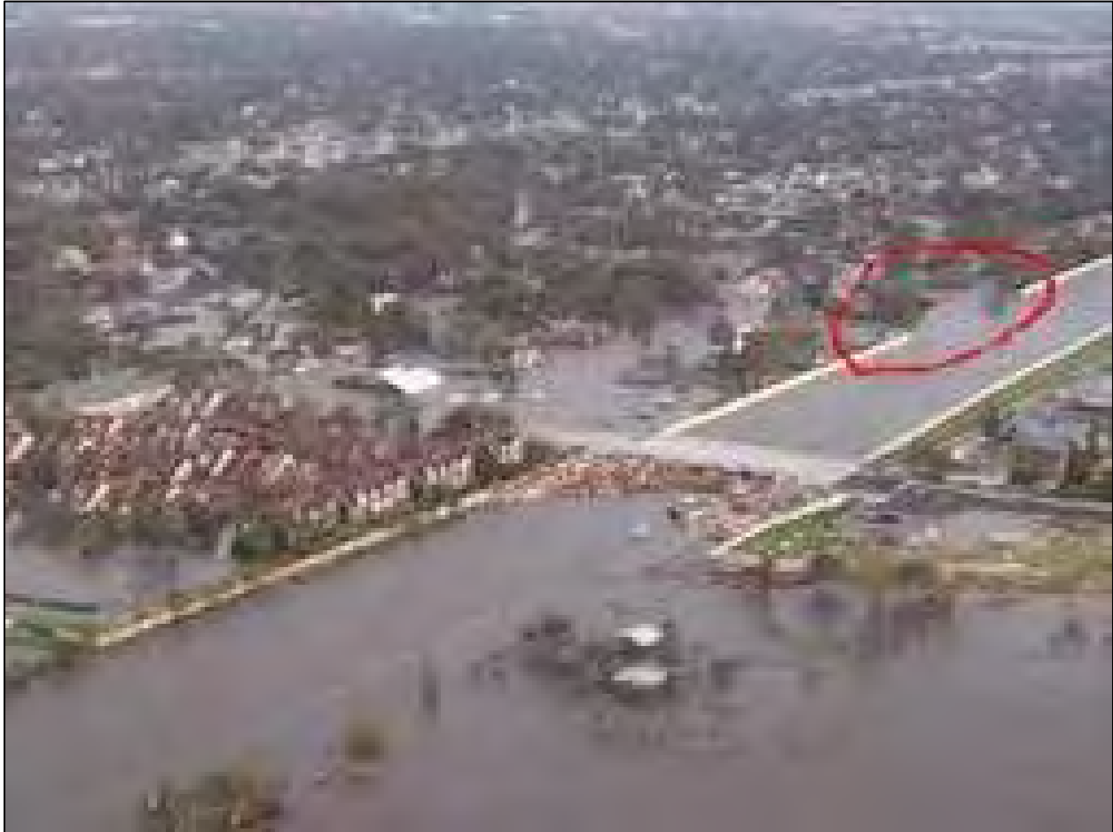
Figure 143. 17th Street Canal August 29, 2005. Looking south showing breach and debris accumulated against lake side of Hammond Highway Bridge
