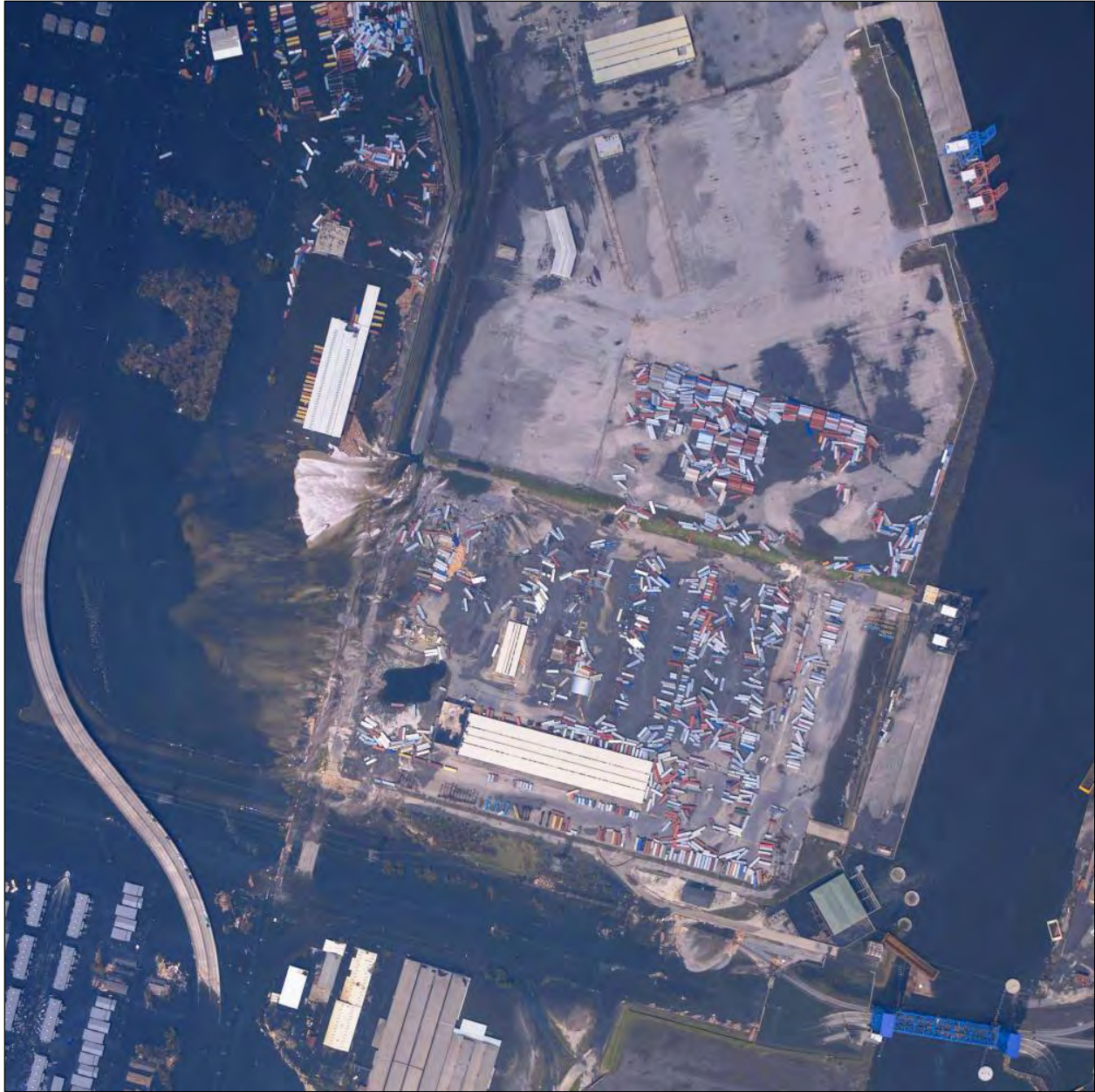
Figure 127. Floodwall and earth levee breaches on west side of the Inner Harbor Navigation Channel.
