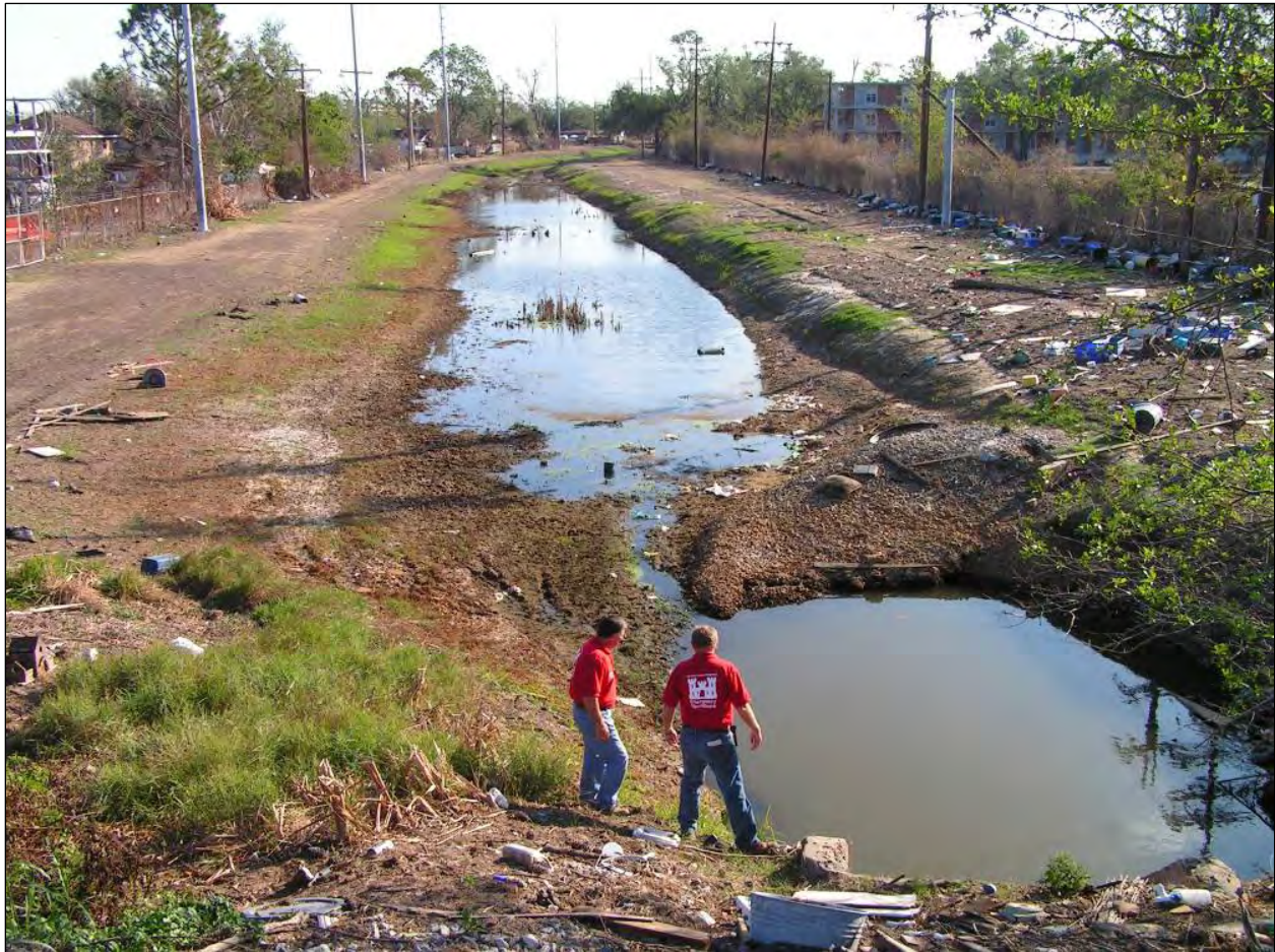
Figure 131. Scour hole east of railroad grade indicating flow from Peoples Canal into the Bartholomew Golf Course area
