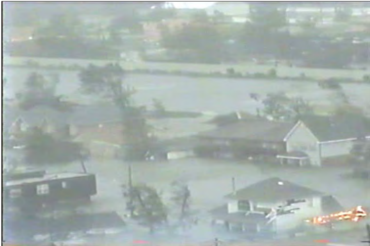
Figure 119. This video frame shows the breach in the 17th Street Canal floodwall and flooding in Lakeview about 11:20 a.m. on Monday, 29 August 2005. The portion of the breach shown in this image is near the intersection of Bellaire Drive and Stafford Place. (Video provided by National Geographic Television)
